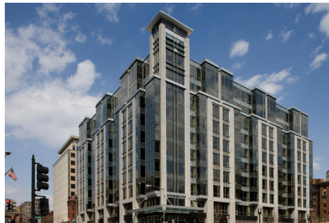
Project: 1101 K Street NW Location: Washington, DC
