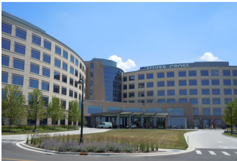
Project: Silver Cross Hospital Location: New Lenox, Illinois
