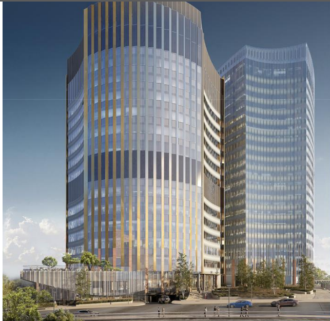
Children's Hospital of Philadelphia Harmon curtainwall Viracon glass
