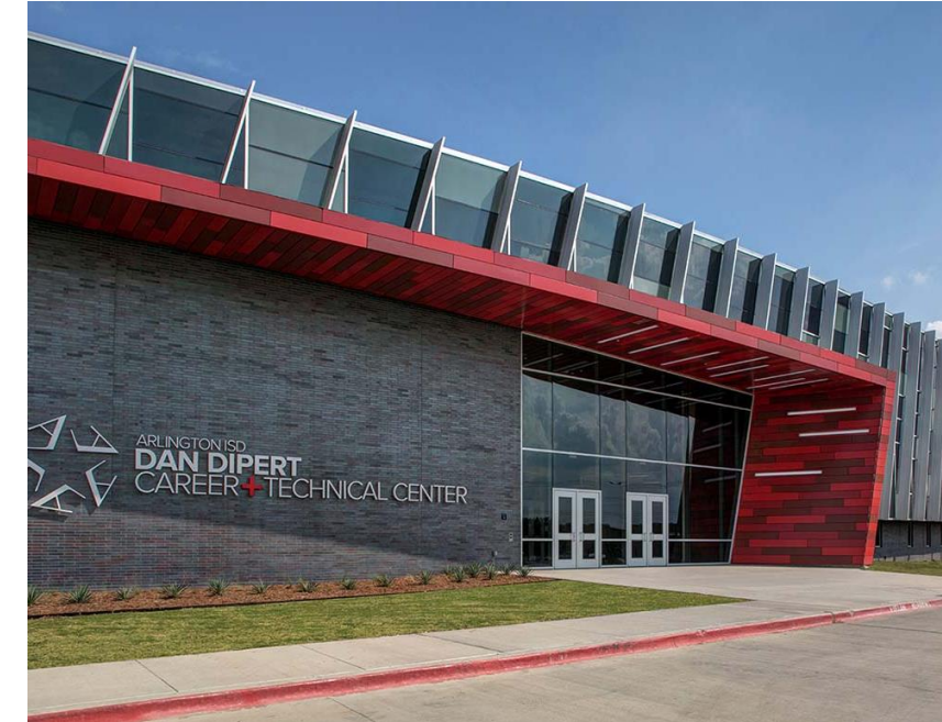
Dan Dipert Career & Technical Center, Arlington, TX Tubelite storefront and curtainwall, Lineteq finishing
