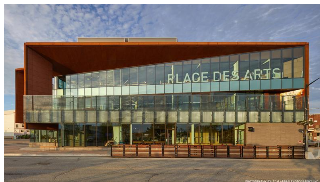
Place des Arts, Sudbury, Ontario Alumicor framing systems Viracon glass
